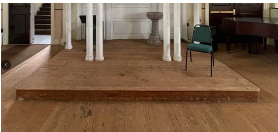
Photograph of existing stage, front portion to be removed and chamfered as illustrated in detail 3/A600
